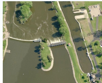
Stratton-Bolger Lock and Dam on Fox River, McHenry County, IL
