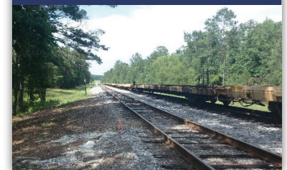
Fort Polk Railroad Rehabilitation, Vernon Parish, LA
