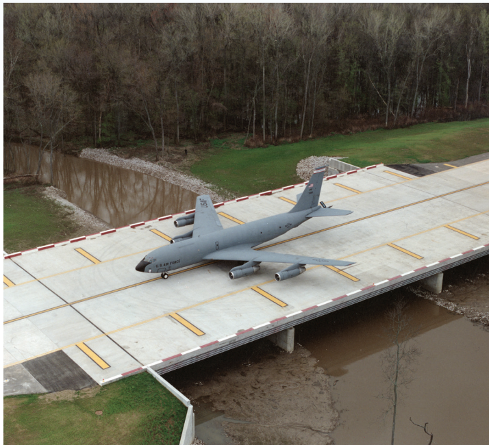
Scott Air Force Base Taxiway Bridge, St. Clair County, IL
